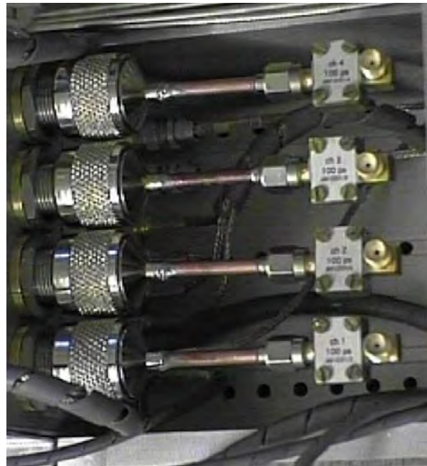
Figure 6 100ps modules fitted
